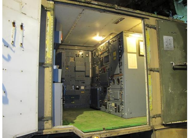
First task – get the lights on!
